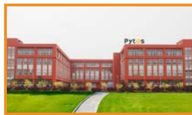
Shandong PYTES New Energy Technology
