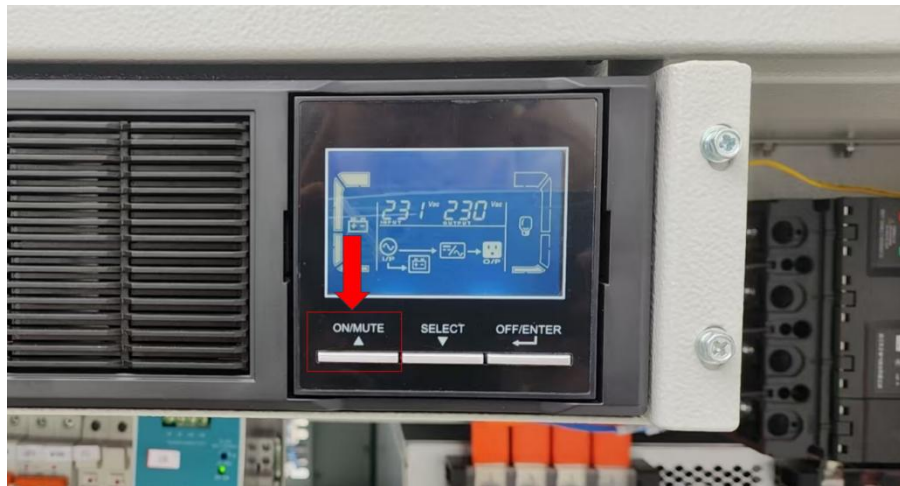
Figure 6.5 Turn on the UPS
