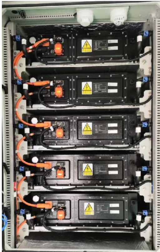
Figure 7.11 Installation Status of Battery Clusters
