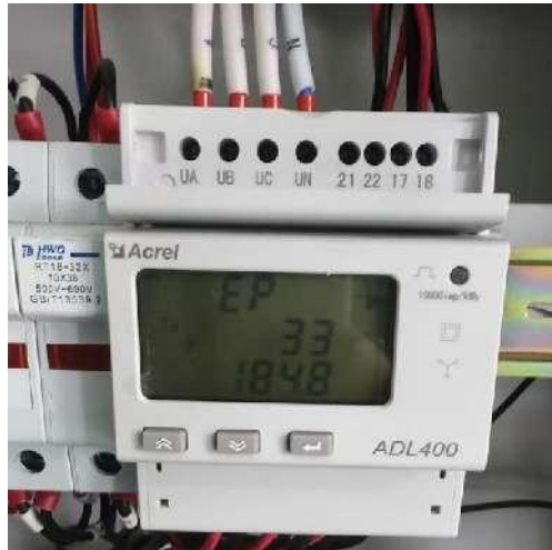
Figure 5.17 Diagram of Electrical Meter Port
