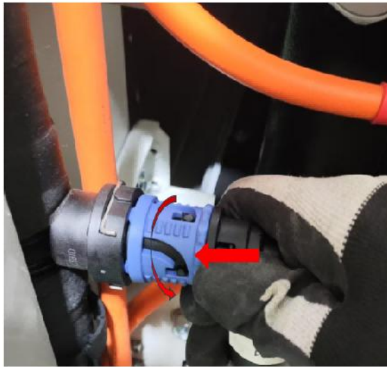
Figure 7.8 Disconnecting the water pipe connection
