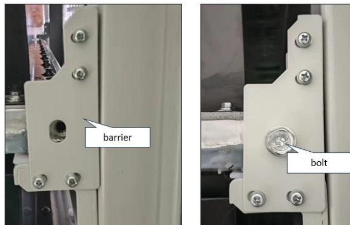
Figure 7.9 Bolt and Damper Plate
